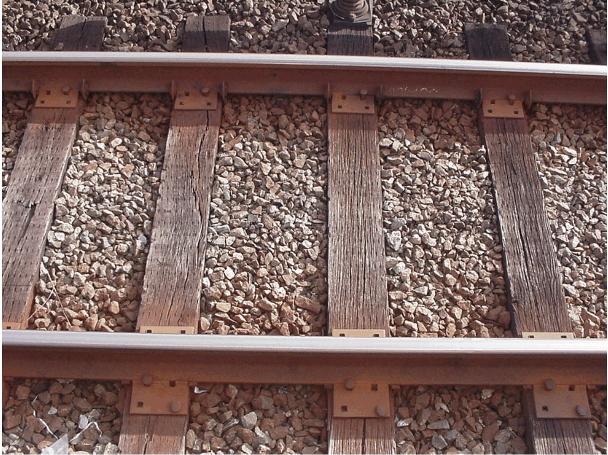
Ballasted Track, Cheverly Station
