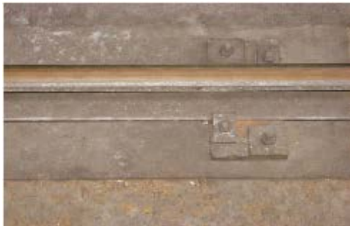
Landis Fastener - Plan View
