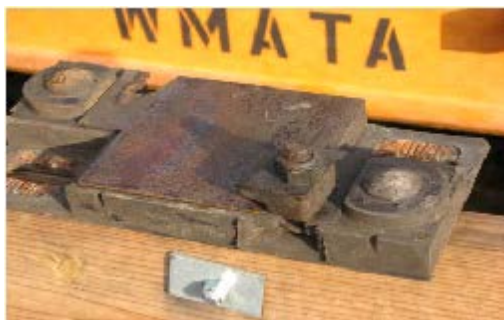
Hixson Fastener - Plan View
